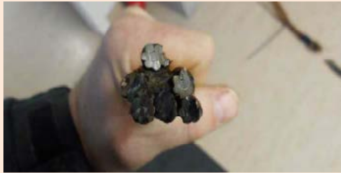
Fibre core wire rope in very poor, corroded condition
