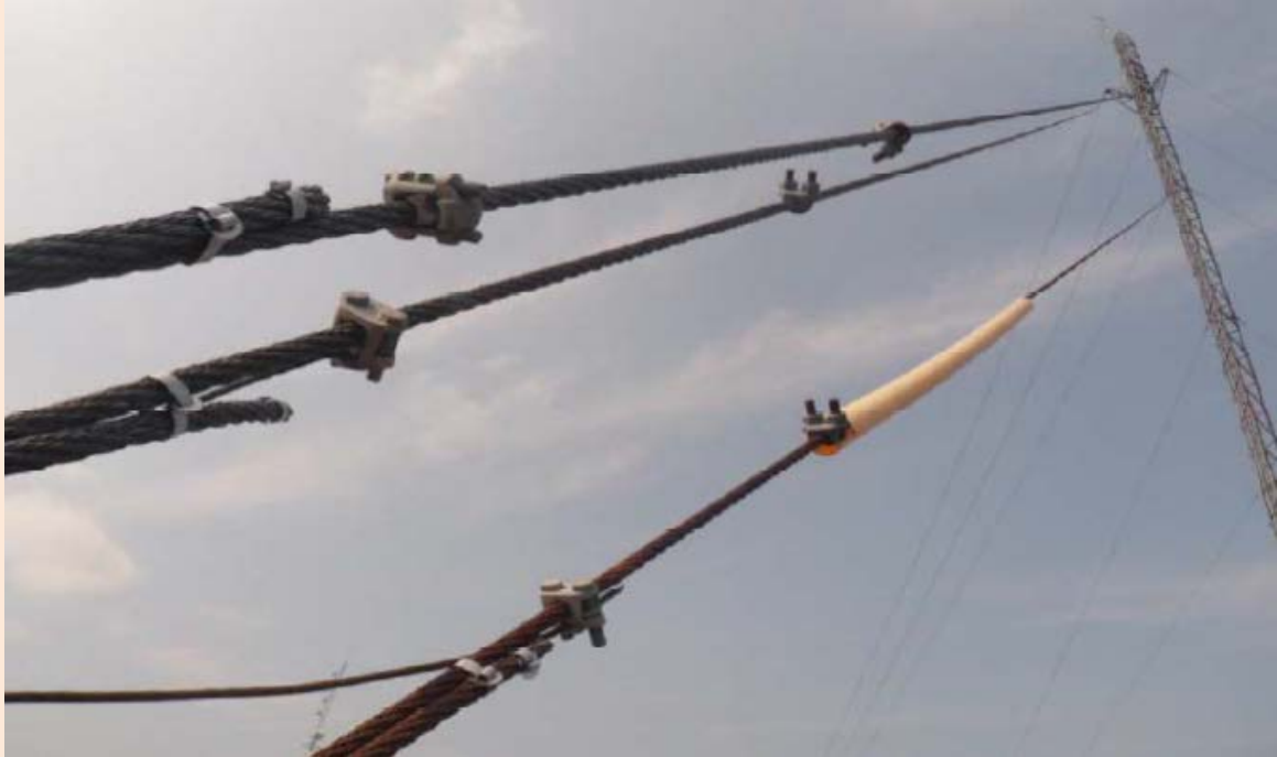
Wire rope guys at the anchor
